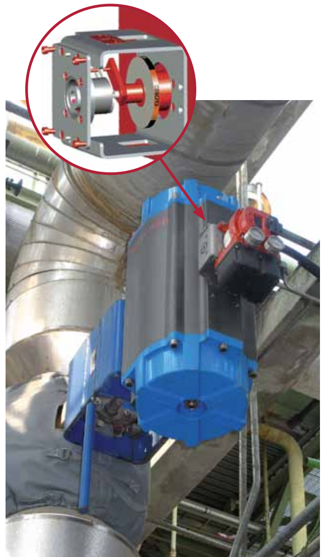
SVI II ESD operating on a quarter turn ESD valve with NAMUR VDI/VDE 3845 mounting kit
